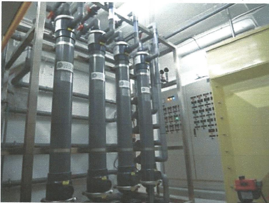
Photo for 100 cu.M per day system – membrane
